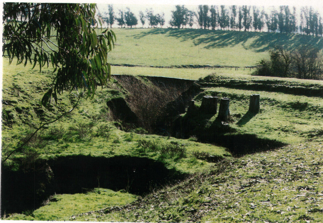
Photo 4. Looking downstream at the failed dam. Note the deeply incised channel.
